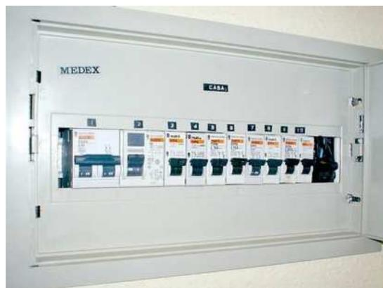
The switch box contains the **general switch** of the installation, which gives input to the electric current to the house circuit, in addition to a series of small automatic switches (**PIAs**) that limit the available power (**limiter**), protect from current leaks (**differential**) or protect the different appliances (kitchen and oven, washing machine, lighting, power sockets, etc.) when there are voltage peaks (excess of electric energy).
